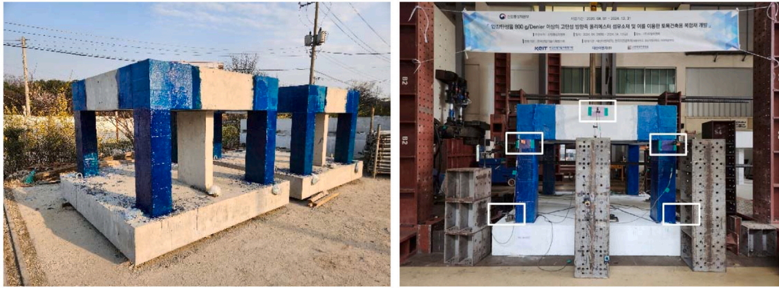
Fig. 5. Installations and test setup of the piloti structures.
